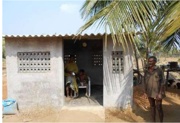
New shelter constructed for him to stay better
